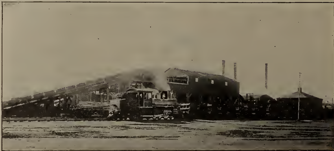
COLLIERIES AT WESTVILLE, NOVA SCOTIA.
